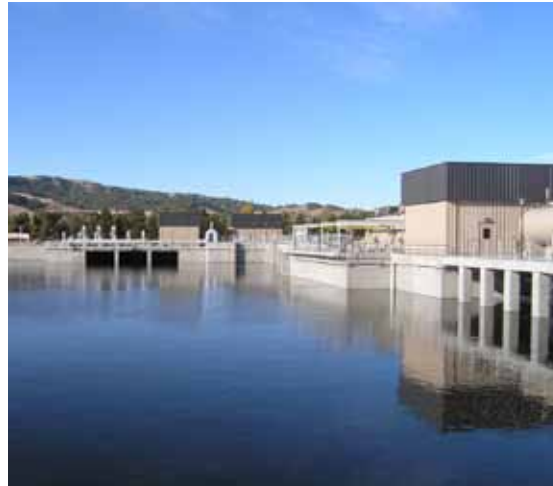
The SRVRWP water recycling plant.
